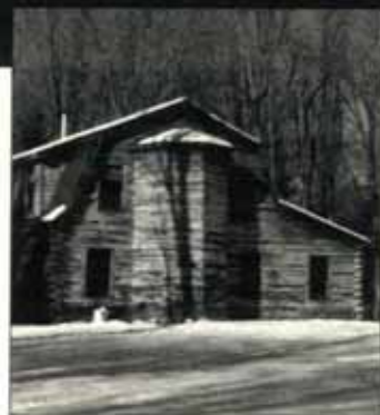
When a cabinetmaker builds a log home, expect some sophisticated joinery. The silo contains a hand-built spiral staircase.
