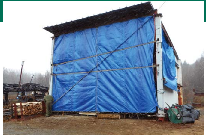
The mill is housed in the sawdust shed of the old mill. The fire heat deformed some of the metal sides, but the roof is sound. The open east side is temporarily covered with a tarp. At the left is a rack sized to hold 1/3 cord of slabs that are banded and sold for firewood. The remains of the old mill are in the left background.
