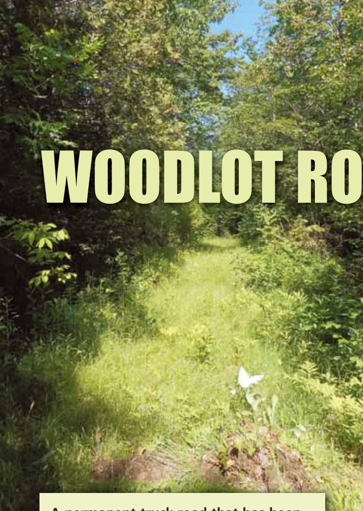
**A permanent truck road that has been graveled, properly drained and seeded, and provides access for logging, hunting, snowmobiling, ATVs and equestrians. Maintenance has been by farm tractors using 3-point-hitch grader blades to maintain drainage, and sickle-bar and rotary mowers to control vegetation.**
