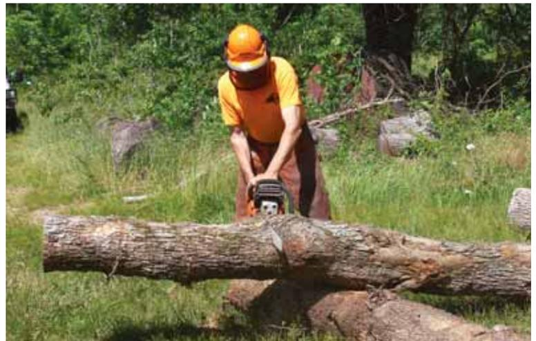
For bucking cantilevered logs without splitting them, first cut the bottom 1/3 of the log; then finish cutting the cantilever log from the top. If you're not sure which way the log is stressed, drive a wedge into the top kerf as soon as you have cut enough room for it.
